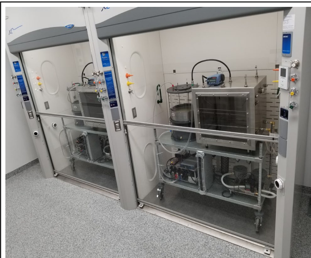
FIGURE C: Inhalation Facility 2.0 Exposure Hoods in the nanomaterial exposure room. Walk in hoods have an airflow pull rate of up to 150 CFM, and can be purged directly to the filtered exhaust system of the facility's HVAC system. Internal aerosol generation/characterization equipment is networked and can be controlled immediately in the room or remotely over the HSC network..
